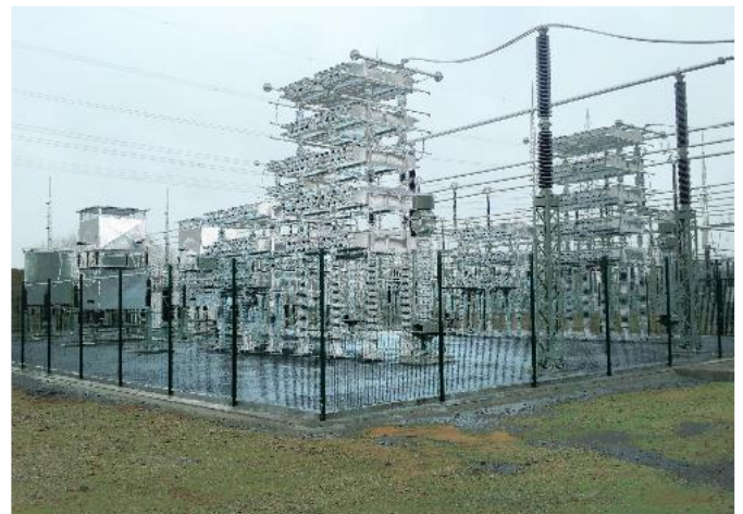
MSCDN installed in Germany
