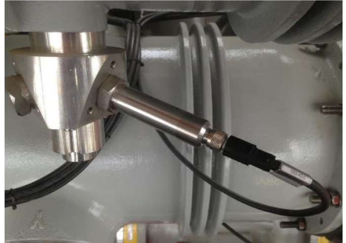
BWatch Integrated SF 6 and g 3 Monitoring System and Internal arc localization for GIS/GIL
