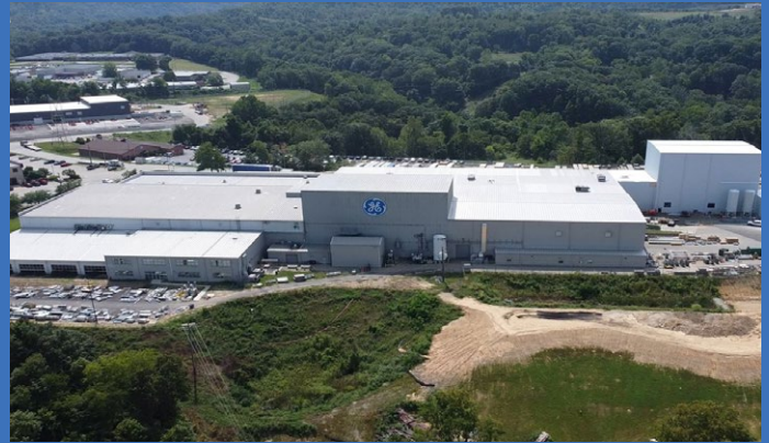
Charleroi Dead Tank Circuit Breaker Center of Excellence
