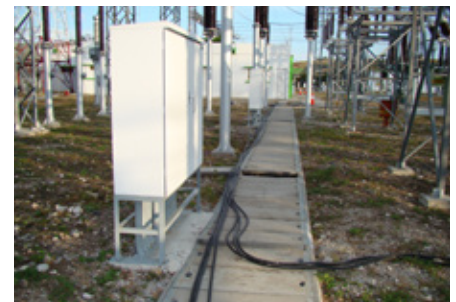
Simple fiber optic cable installation
