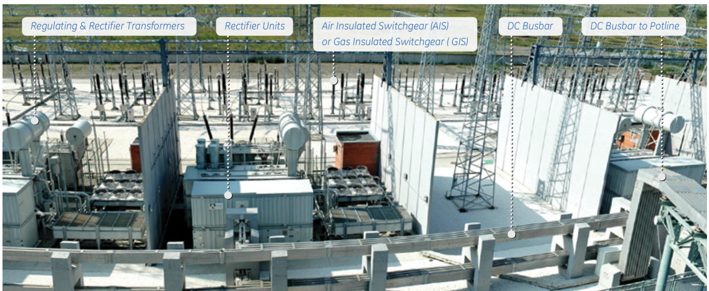
Typical DC System - Aluminium Smelter Conversion Substation
