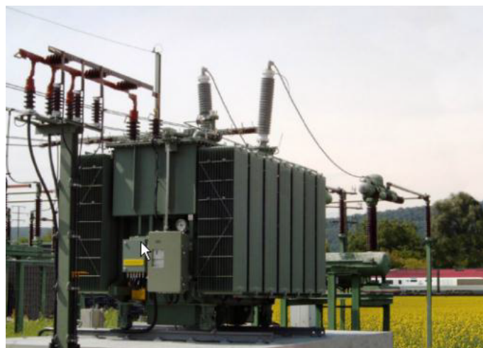
Fig. 2: Hermetically-sealed power transformer
