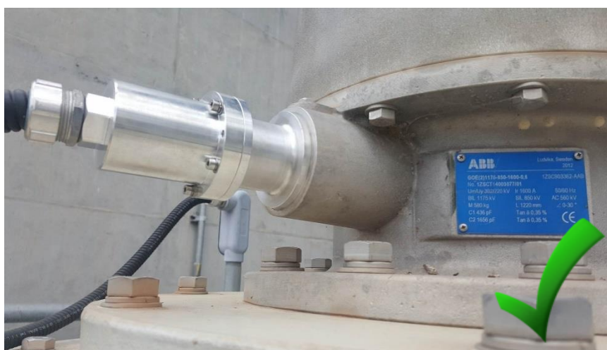
Figure 11-12: Bushing adaptor installation – good example
