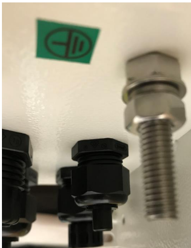
Figure 8-2: Position of primary protective earth bonding lug
