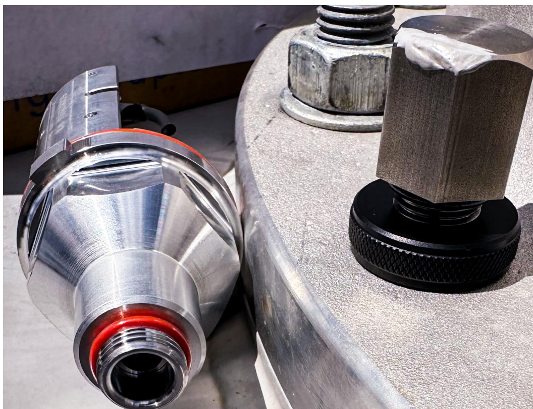
Figure 11-11: Bushing Adaptor with original test tap cover – thread check
