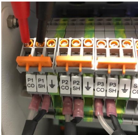
Figure 11-76: Input voltage measurement
