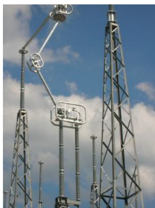
SPVL Semi-pantograph disconnecter
