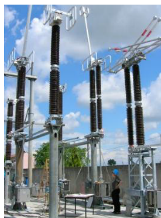
S3CVL Vertical break disconnecter
