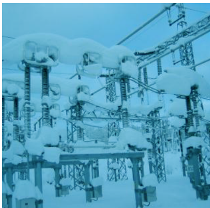
An SPOL 300 kV knee type disconnector equipped with L-Contact in extreme weather conditions in Norway
