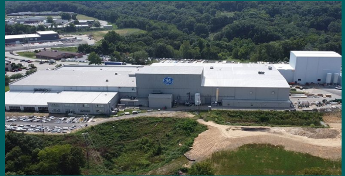
Charleroi Dead Tank Circuit Breaker Center of Excellence
