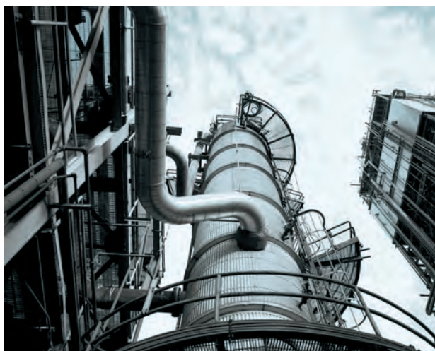
Figure 7. integrated coal gasification combined cycle (IGCC) power plant
