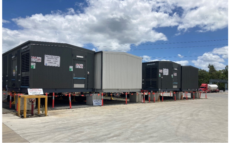
Buildings can be constructed and tested off-site in advance, enabling deployment when the site is ready
