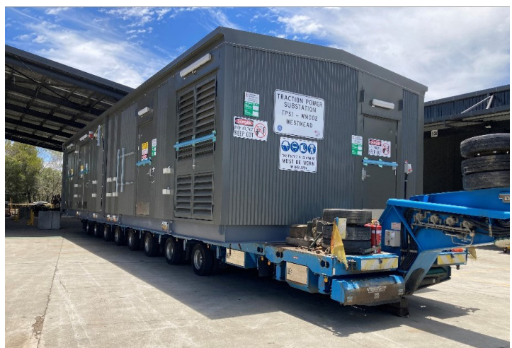
Off-site traction power substation construction
